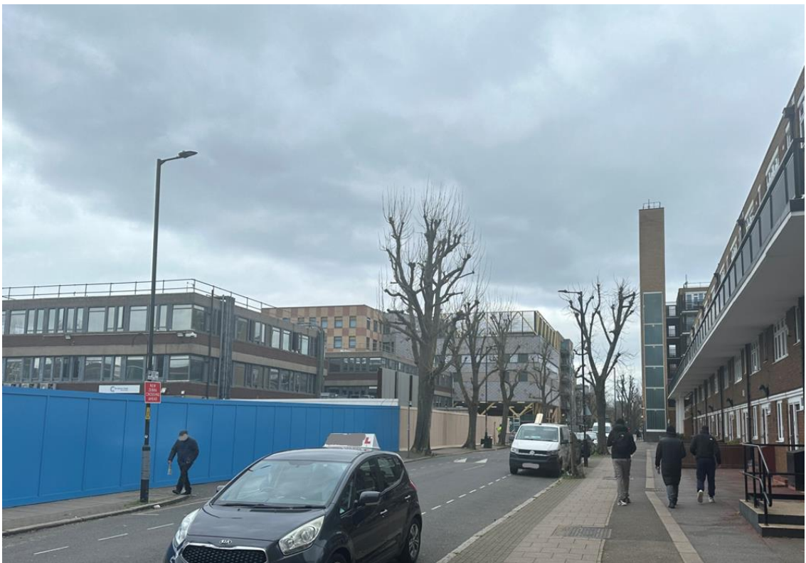
View looking north on Drummond Road to block 1-4 and new school
