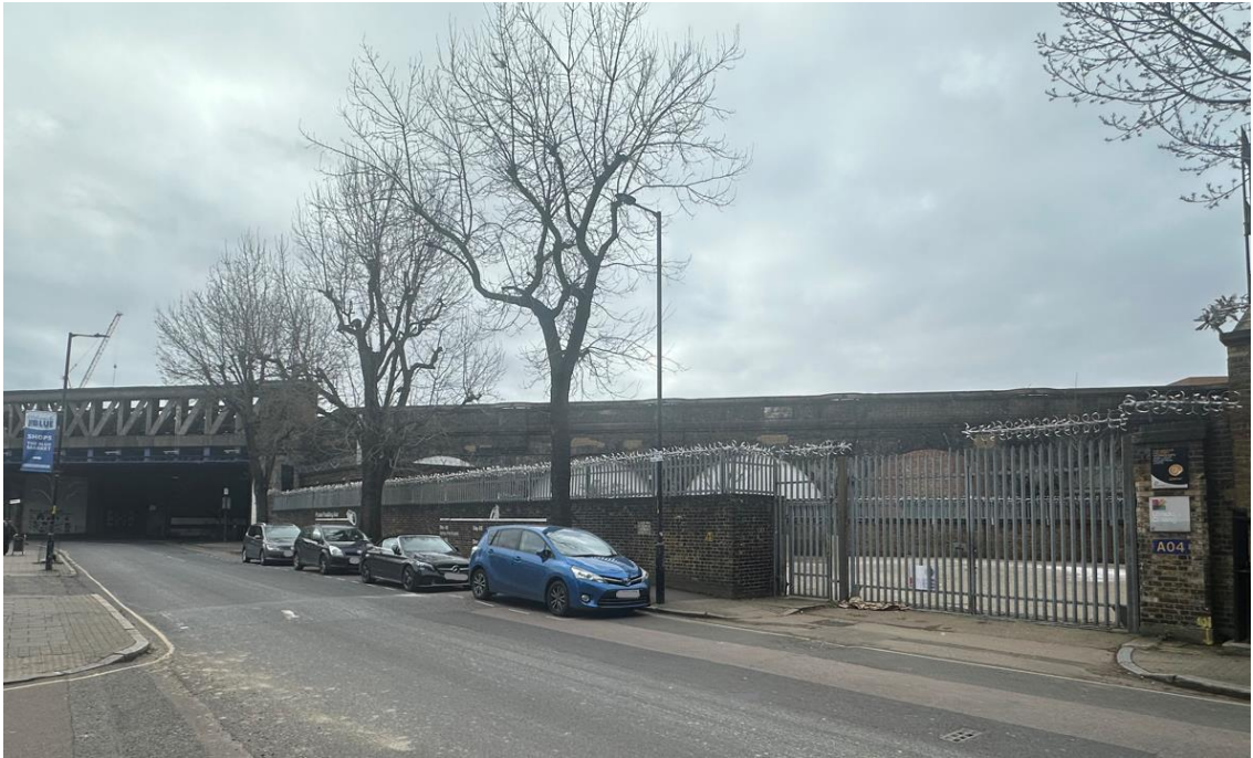
View looking south on Drummond Road to the yard where block W is proposed and the railway viaduct
